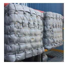
New Componit PFP consists in flexible jackets to be directly installed on valves or actuators and any kind of equipment that need to be protected from fire for safety reasons.
