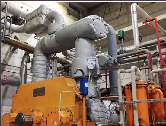
Piping and turbine
