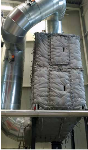
Insulation for SCR
