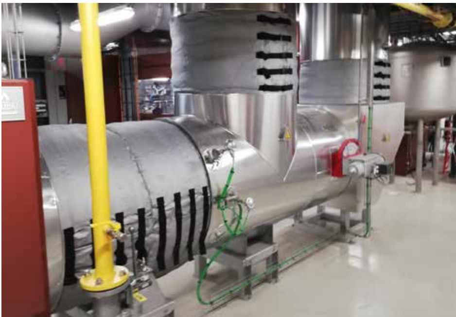
Insulation for food plant
